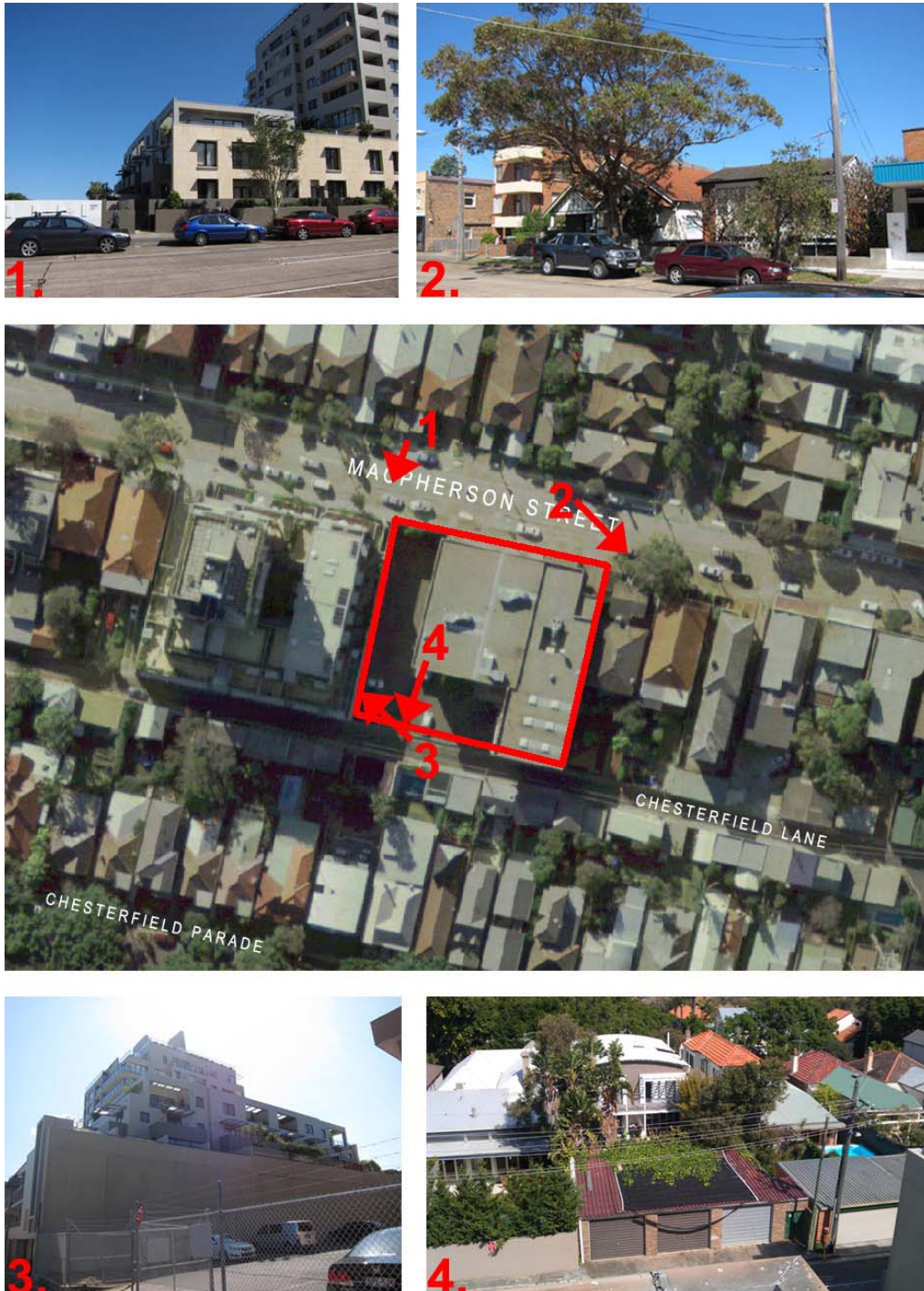
Figure 7: Views of Streetscape, Townscape and Built Form Character Adjoining Site
